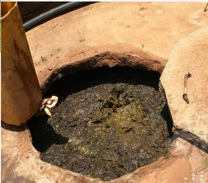
Biogas plant at the KHEA multiplier's farm. Slurry got from cowdung is used in production of biofertilisers
