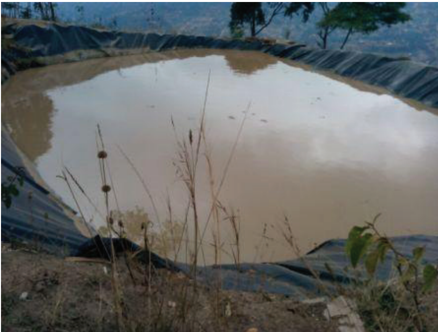
A polythene lined dam for harvesting rainwater run off constructed by Zipporah Wambua
